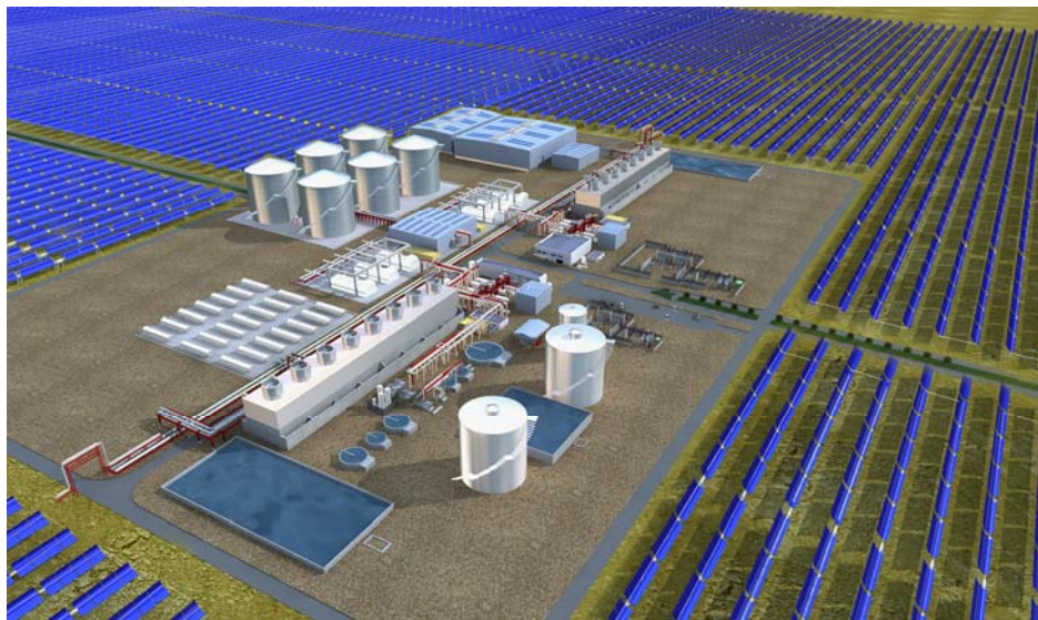
Figure 6: Schematic of the Solana CSP Plant Power Block
