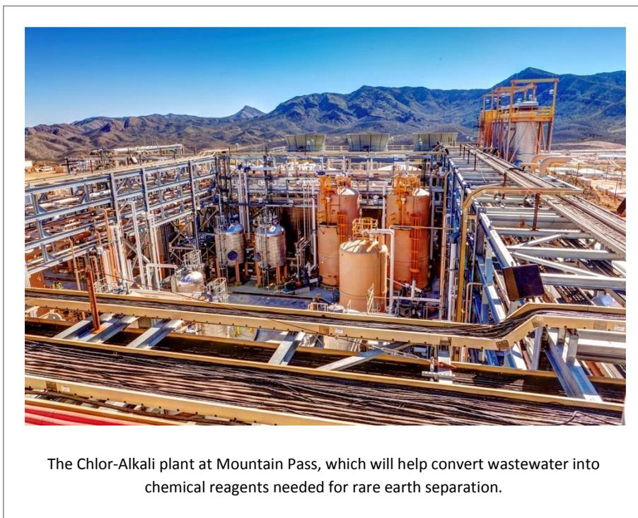
The Chlor-Alkali plant at Mountain Pass, which will help convert wastewater into chemical reagents needed for rare earth separation.
