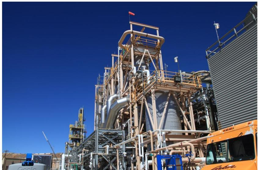
collection of 12 operating systems that must work together both in series and in parallel. As our current rare earth production ramp-up continues, we are working to optimize and strengthen the system, improve rare earth recovery rates, improve on-time reliability, add redundancy, and increase product throughput.
