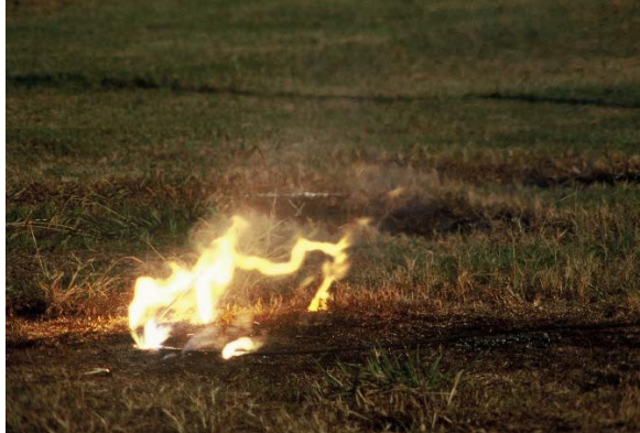
Figure 2: Downed line arcing
