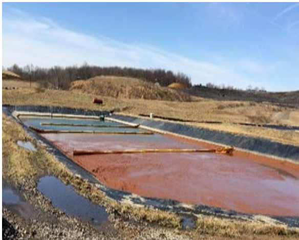
Figure 1. Typical AMD sludge settlement cells at a Pennsylvania coal mine. The orange material in the foreground is enriched with rare earth elements. After the metals precipitate, the clear water in the far cells is discharged via a regulated discharge point.
