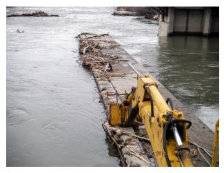
The dam crest was raised probably in the 1980's, but the trash rack was not raised and that allows debris to enter the headgate intakes.
