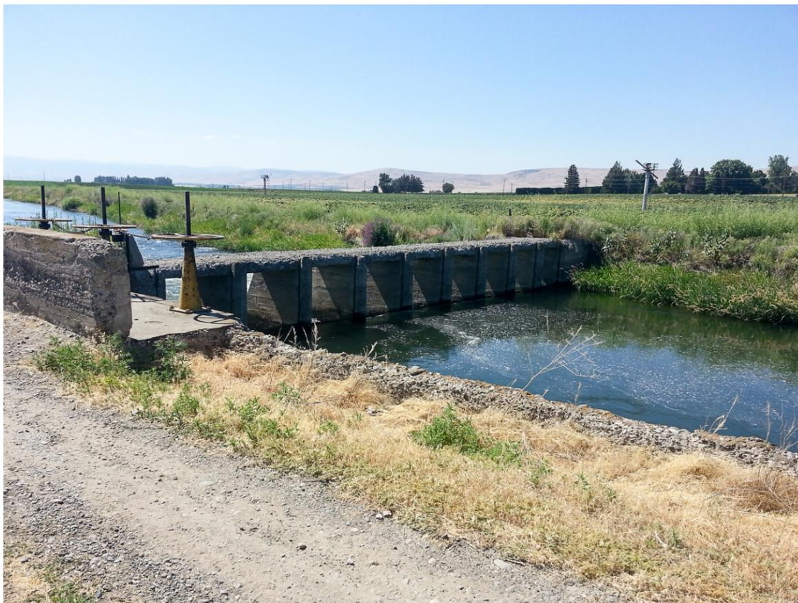
Main Canal Check Structure for Lateral 2 & Drain 2.
