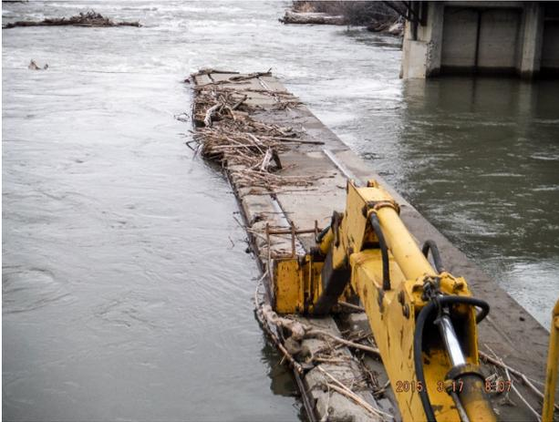
The dam crest was raised probably in the 1980's, but the trash rack was not raised and that allows debris to enter the headgate intakes.
