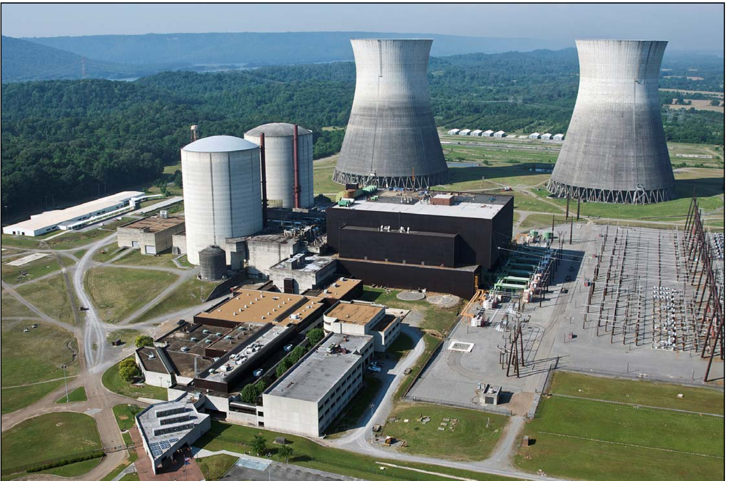
Bellefonte Nuclear Plant Unit 1, Alabama
