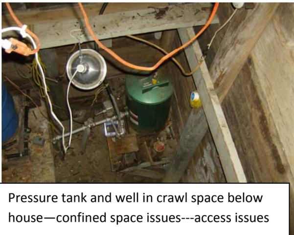
Pressure tank and well in crawl space below house—confined space issues---access issues
