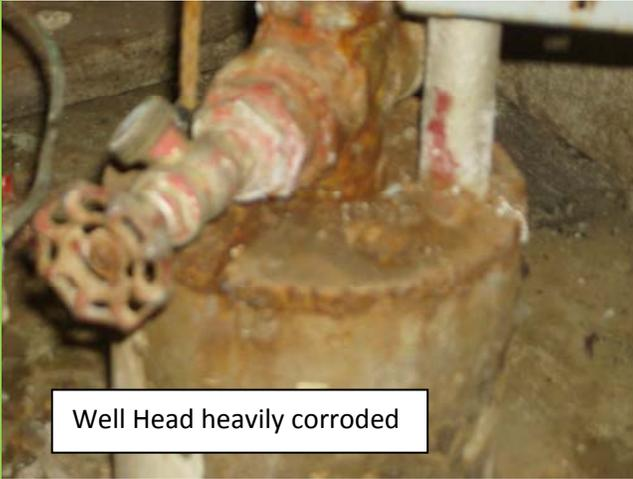
Well Head heavily corroded
