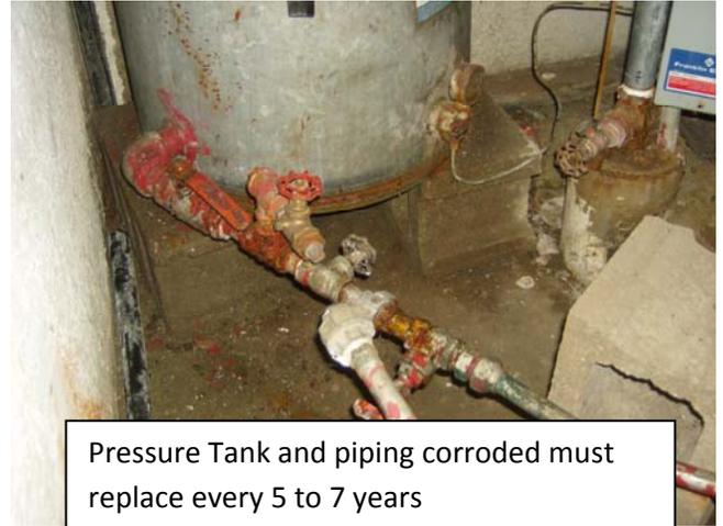
Pressure Tank and piping corroded must replace every 5 to 7 years
