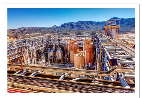
The Chlor-Alkali plant at Mountain Pass, which will help convert wastewater into chemical reagents needed for rare earth separation.
